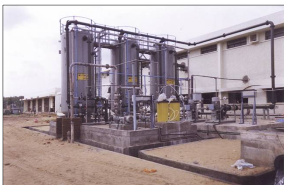
1800 cubic metre Reverse Osmosis based desalination plant at Kalpakkam
