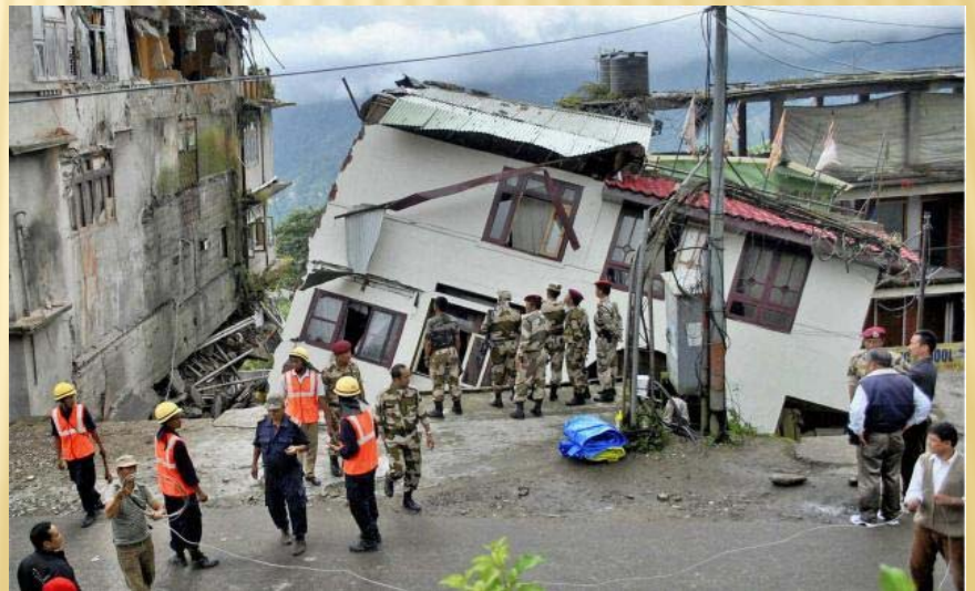
Social Infrastructure: Damage to houses
