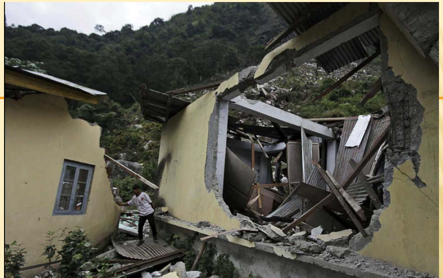
Governance Infrastructure: 1255 nos Government buildings damaged
