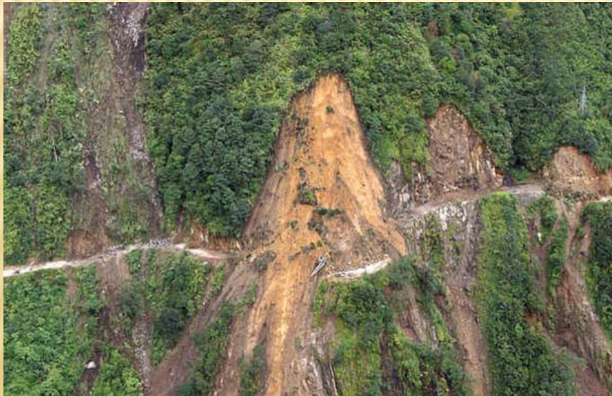
Transport Infrastructure: Total 3,230 km of roads damaged
