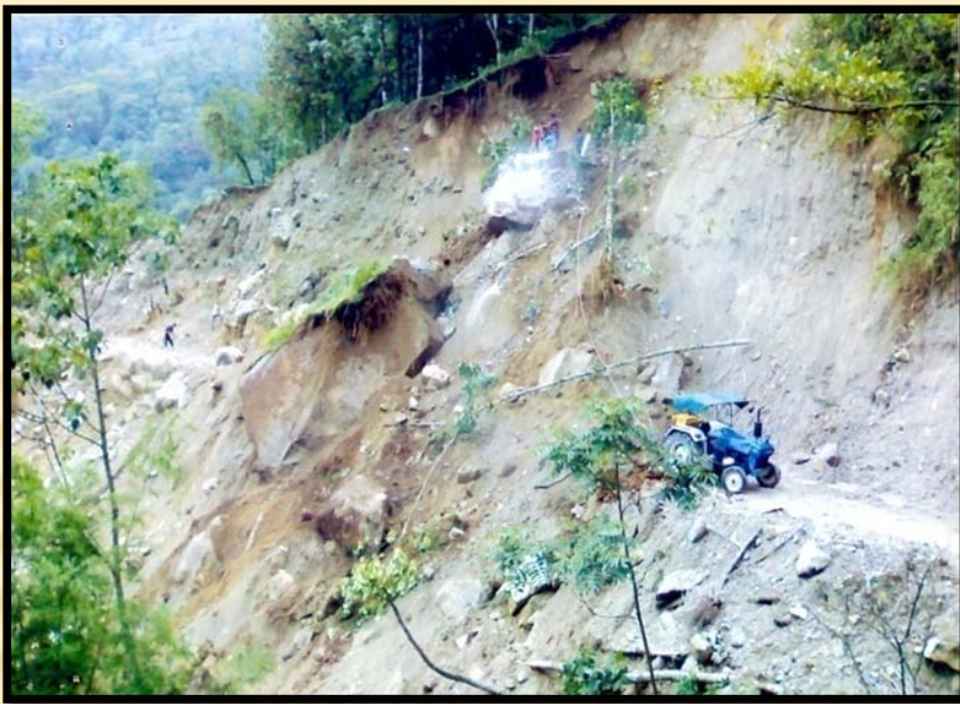
Transport Infrastructure: PMGSY rural roads damaged
