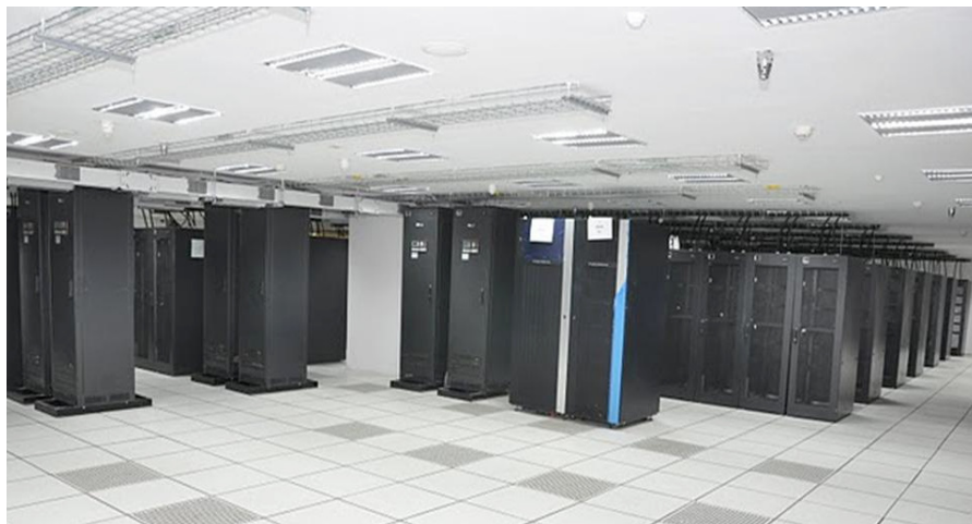
Figure 6.3:View of a Data Centre
