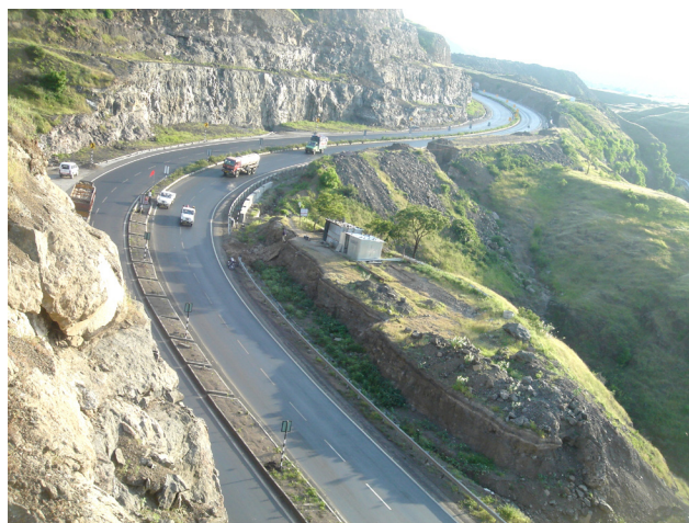
Figure 2.1. Aerial view of one of the highways developed under NHDP
