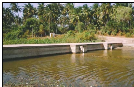
Muthukunder Weir, Block-Chittoor, District-Palakkad
