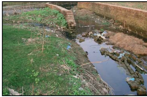
Drainage Constructed by UP Project Corporation
