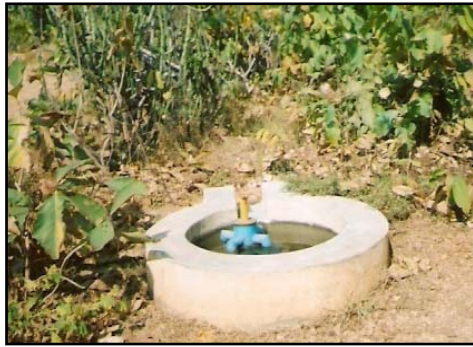
Lift Irrigation Scheme — Outlet Point
