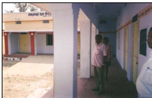
School Building, GP-Jilundi, Block-Bhanjanagar, District-Ganjam
