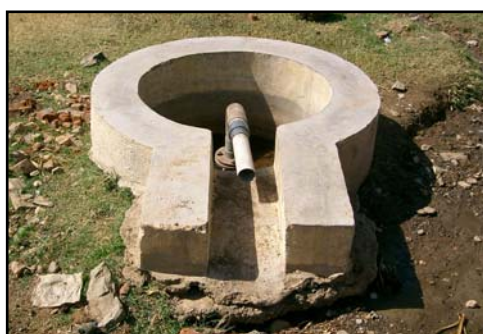
Outlet — Lift Irrigation
