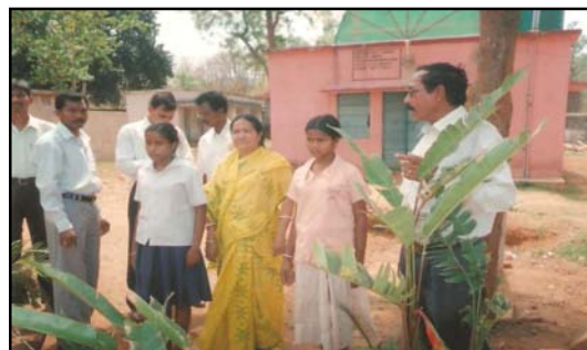
Toilet Complex, Village-Kukudimandi GP- Kulaisila, Block-Rairangpur, District-Mayurbhanj
