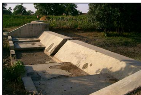
Dry Check-dam in Village Mahuda
