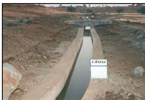
Lining of Canal in Village Kalakhet Goldhar, GP Bawaliyapada
