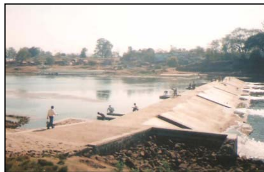
Stop dam-cum-causeway GP-Debra, Block-Dindori, District-Dindori
