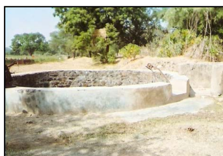
Dry Community Well (Village - Lonawada)
