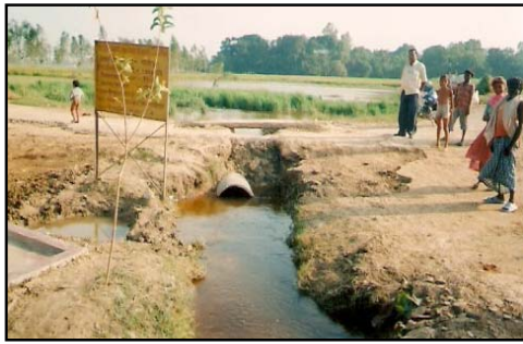
Road Constructed by UP Samaj Kalyan Nigam
