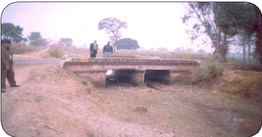
Jewer Distributary at Bridge site at RD 44.0 Km
