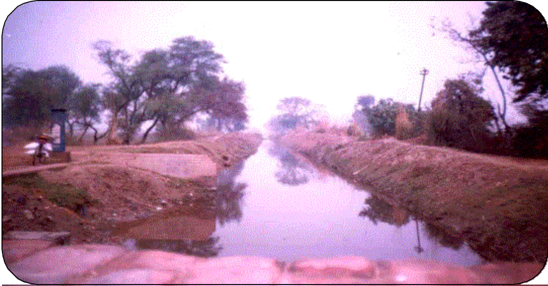
A VIEW OF BALDEO DISTRIBUTARY
